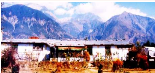
Ningtob Ling began with a temporary hut with tin-sheet roof secured by local stones
